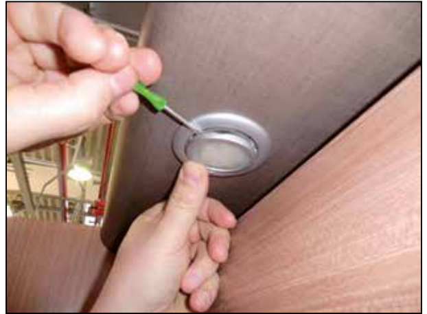
Fig. 91 Replacing lamps of the integrated spot
